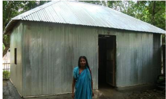
Condition after construction
