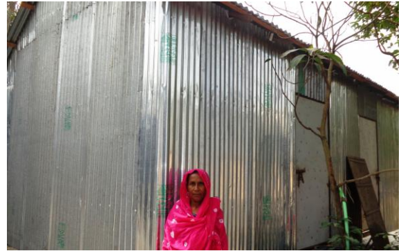
Condition after construction
